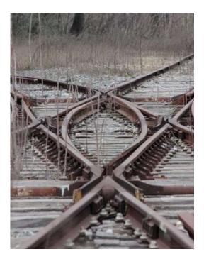
**2.1 Rail System** (Rail, Stock Rail, Check Rail, Frog Rail, Wong Rail, Switch Machine, Fastener, Sleepers and Ballast)
